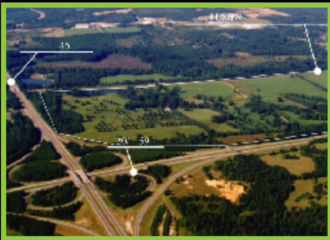
Meridian I-20/I-59 Industrial Park 577 available acres 577 largest tract available Water and power on site Railroad adjacent to site Within 150 miles of three automotive assembly plants (Nissan - Canton, MS, Mercedes - Vance, AL, Hyundai - Montgomery, AL)
